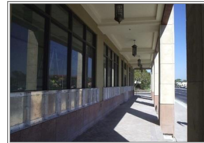
Example of Dry Flood Proofing removable panels utilized in a Bank Building in Naples Fl. – Appropriate in the Bayfront, Entertainment District Core, Neighborhood Crossing, and Town Center Crossing Zones
