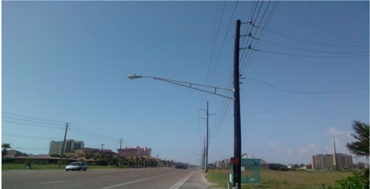
14' Arm with 250 HPS Lighting - (Image of Option 2)
