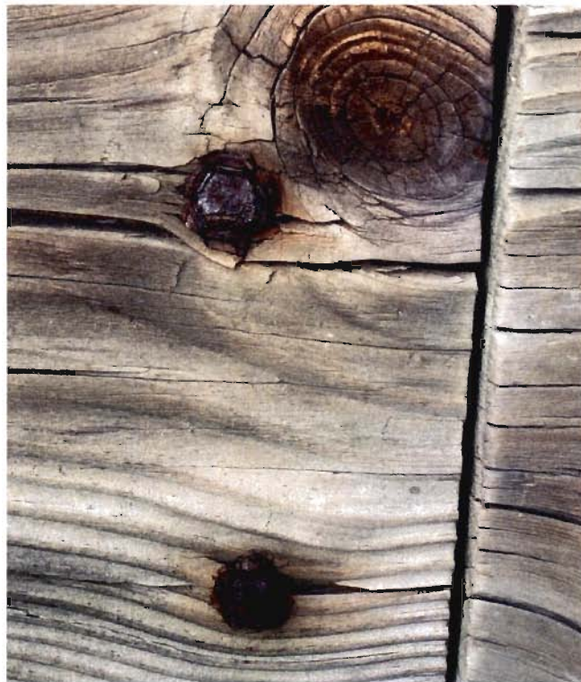
Photo #6 Advanced Nail Corrosion
