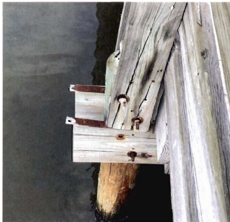
Photo #2 Advanced Splitting at Through-Bolt Connections. Replacement of Guardrail Post Member Shown.
