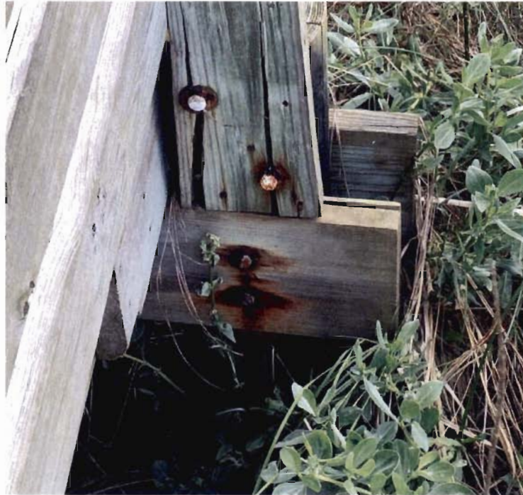
Photo #1 Advanced Splitting at Through-Bolt Connections. Replacement of Guardrail Post Member Shown.
