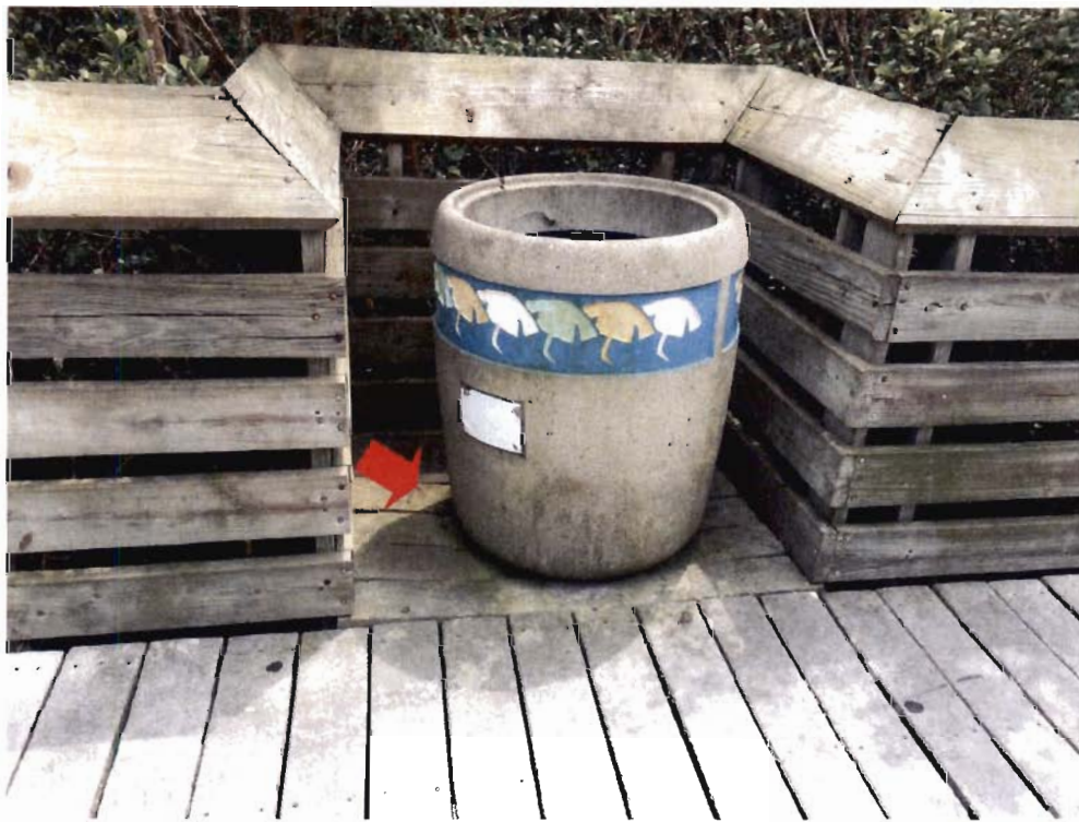
Photo #4 Walking Deck Surface Deflecting Under Trashcan
