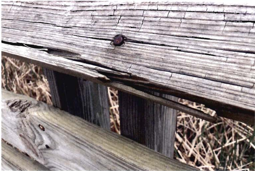
Photo #5 Top Rail Splintering & Advanced Nail Corrosion
