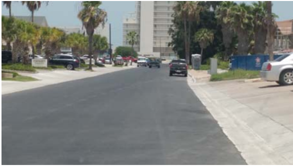
East Atol Street completed.
