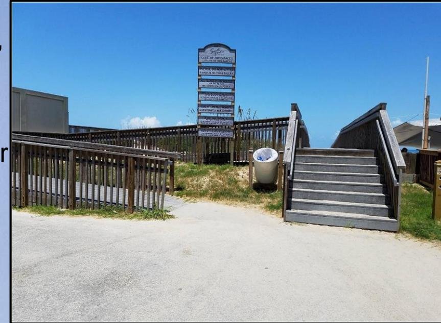
Construction materials: Wood, Trex Planking
