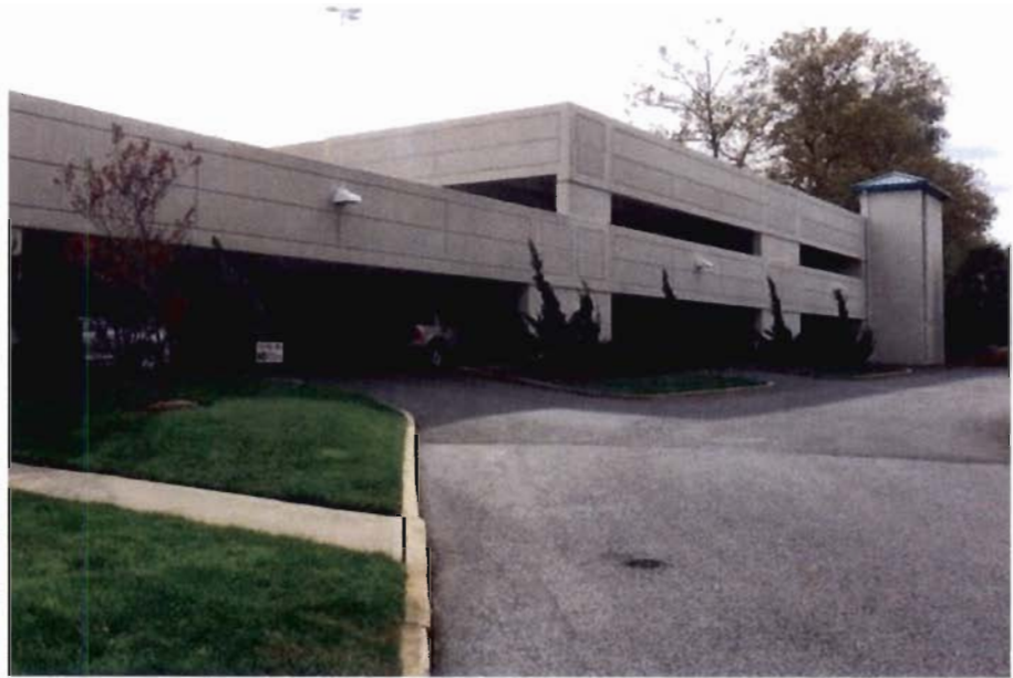
Example of Parking Structure
