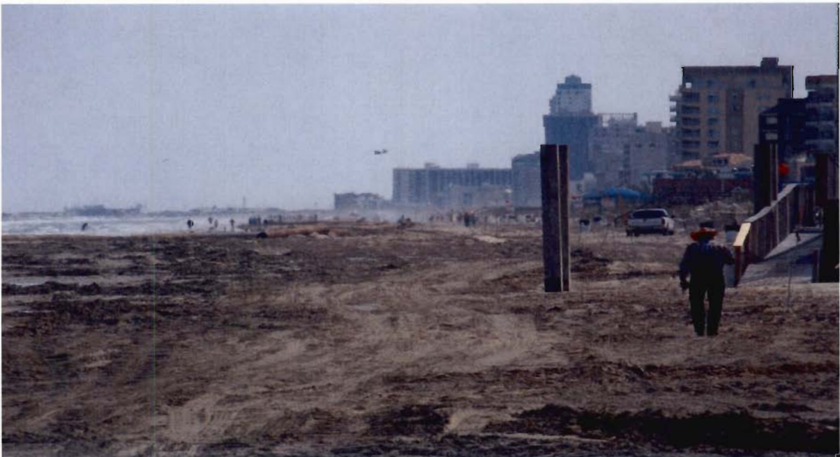
Re-nourishment from Dredge Material
