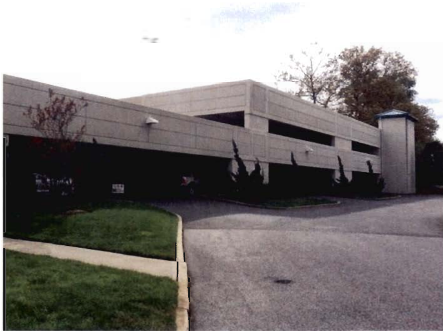
Example of Parking Structure
