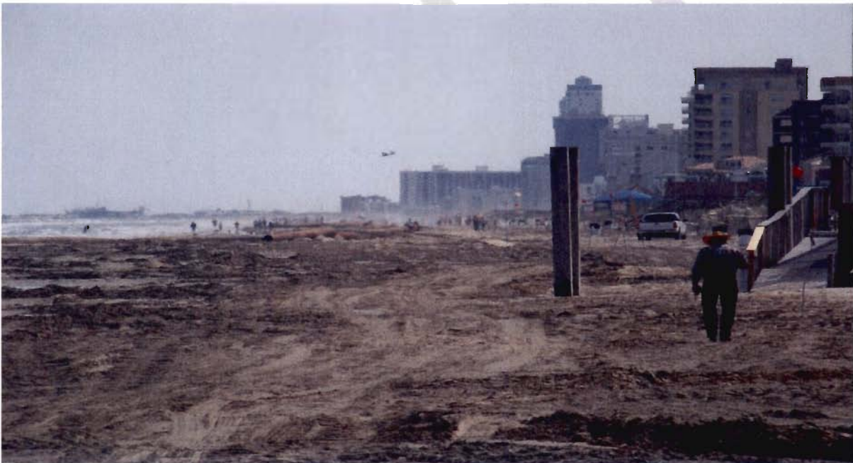
Re-nourishment from Dredge Material
