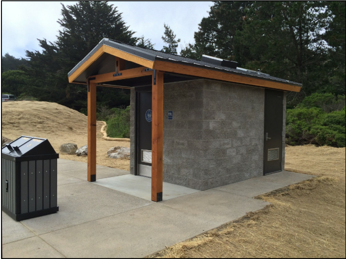
ASPEN WITH PORCH AND ROOF EXTENSION
