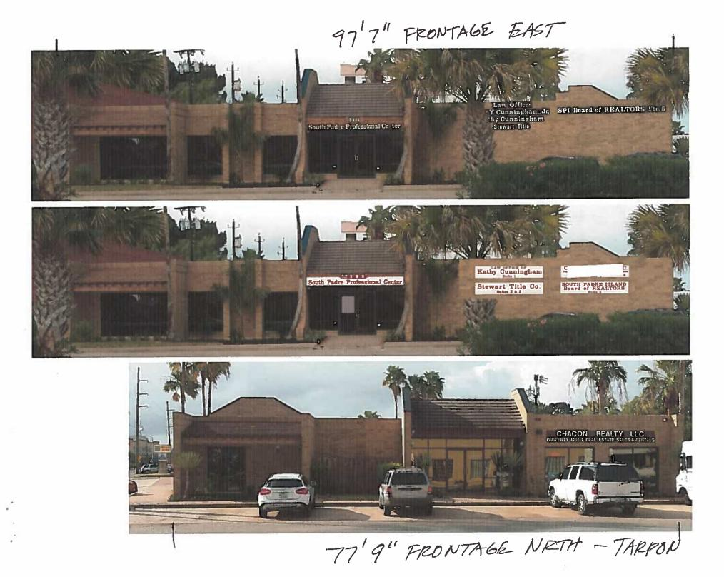
The 3M Vinyl lettered signs are to be made of .063 aluminum with a 1" lip & mounted on 1" aluminum square tubing attached to the brick & cedar wall.
