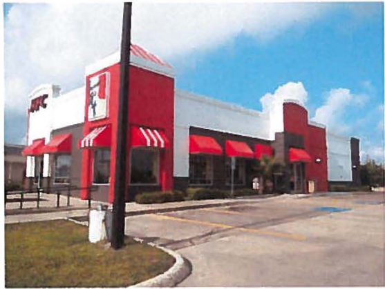
(The existing building)
