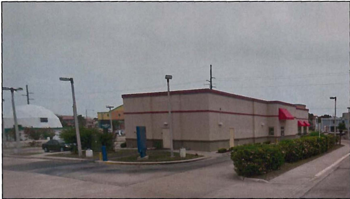
Side of Building Closest to Laguna Blvd.
