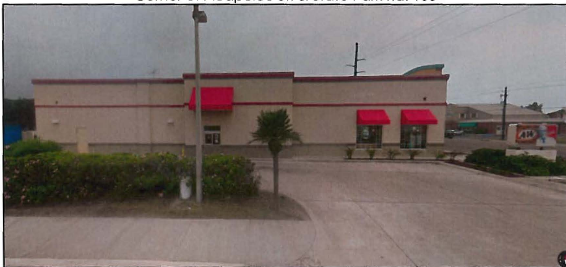
Side of Building Closest to Acapulco St.
