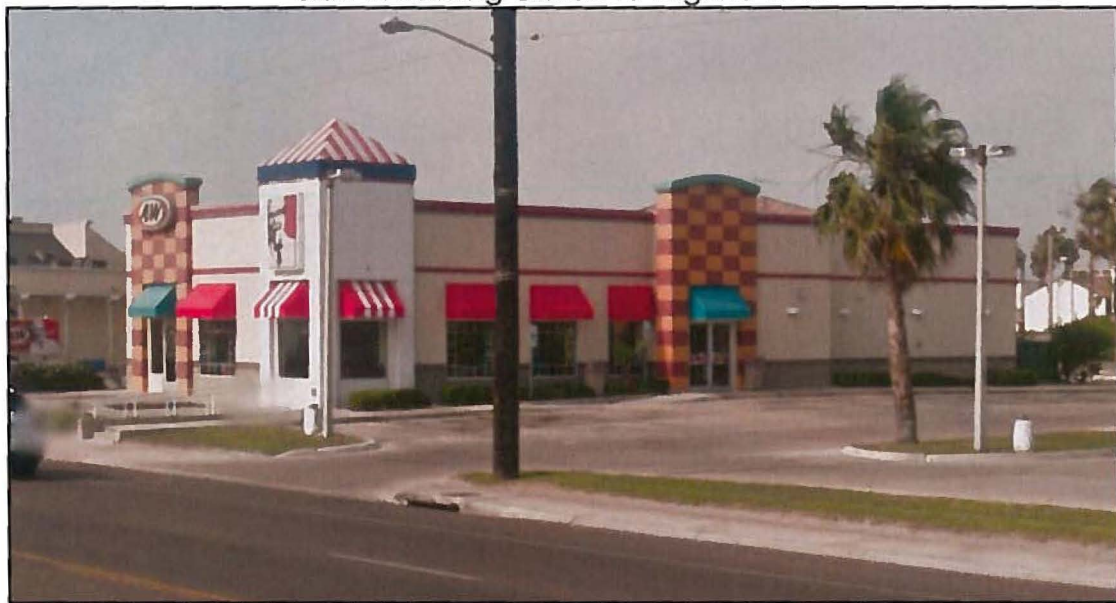
Side of Building Closest to Campeche St.
