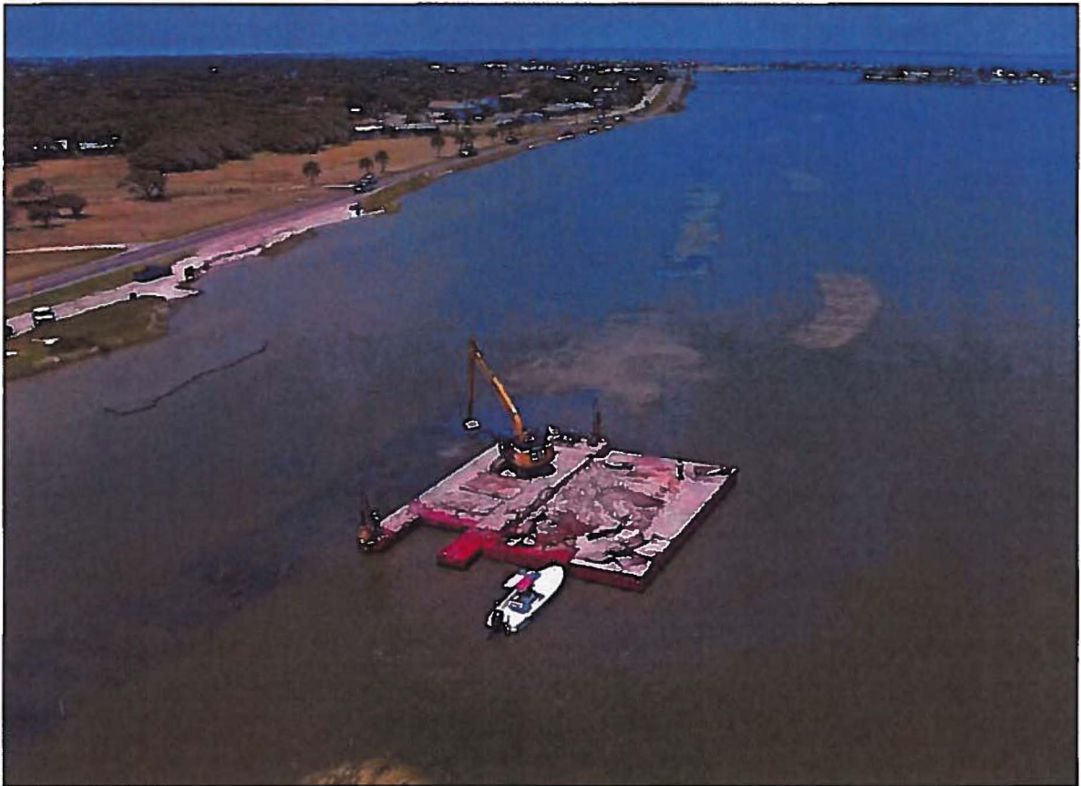
The Live Oak Peninsula Shoreline Stabilization and Enhancement Project in Rockport, Texas involved the construction of oyster reef/breakwaters in order to reduce shoreline erosion and encourage the recruitment and establishment of oysters.
