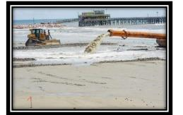
dredge the channels and place the approximate 225,000 cubic yards of sand onto the beach. It will take an additional 7-10 days to remove the tractors and bull-dozers once the project has been completed.
