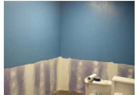
Visitors Center Restroom Remodel Completed 6/1/12
