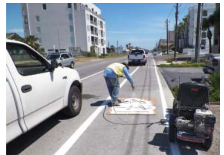
Street & Beach Access Restriping Gulf Blvd. Striping : Completed 9/14/12 Beach Access Striping: Pending
