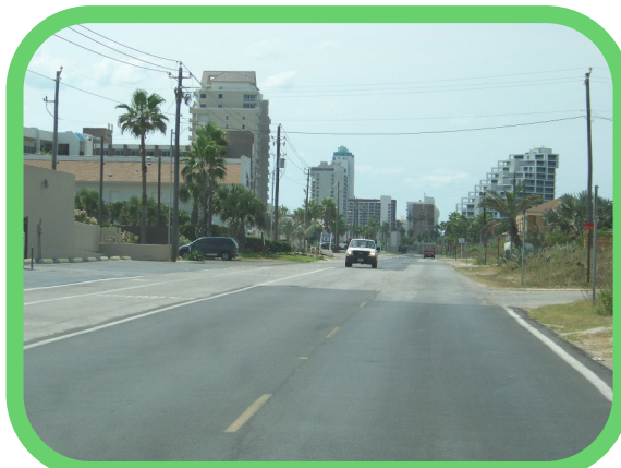
Street Paving Project June 2011
