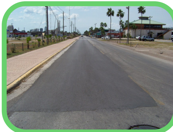
Laguna St. Paving June 2011
