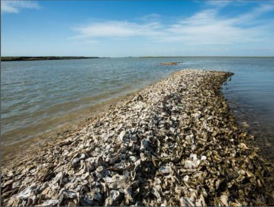
Oyster Breakwater – Jerod Foster & TNC
