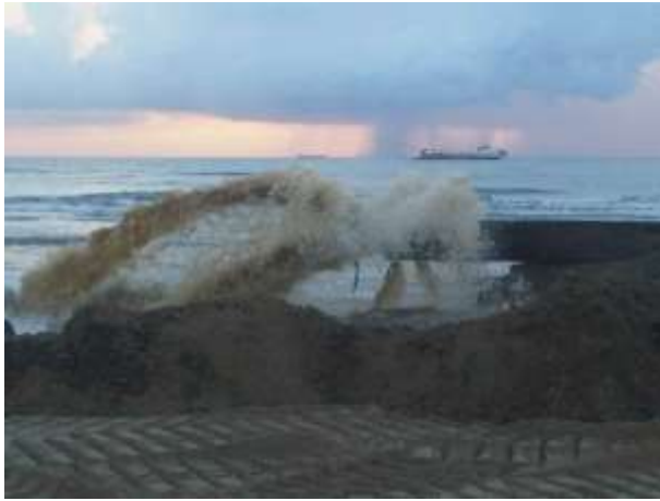
Figure 7. Beach nourishment at South Padre Island using a piped sand/water slurry
