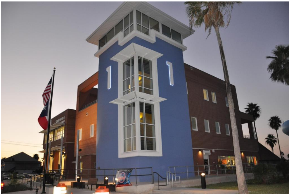
Completed Fire Station
