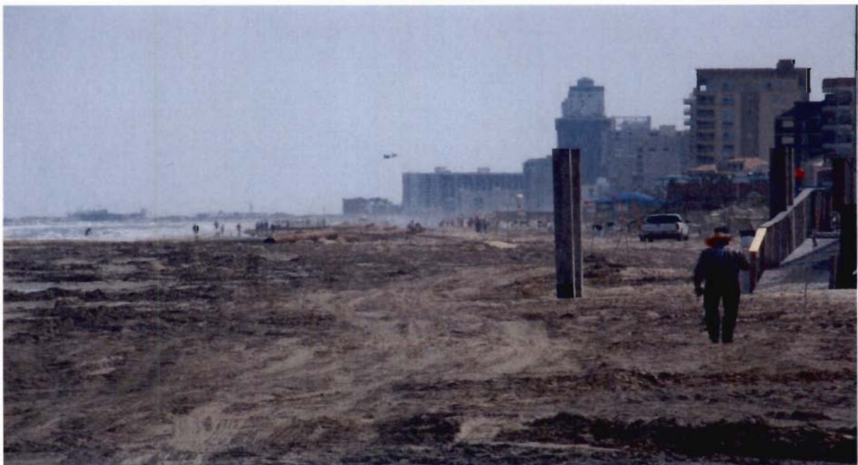
Re-nourishment from Dredge Material
