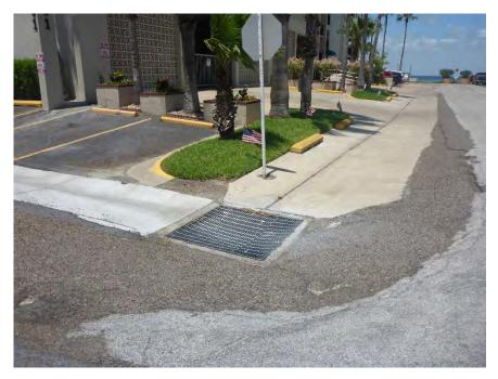
Figure 16. Example Grate Inlet, Laguna Boulevard
