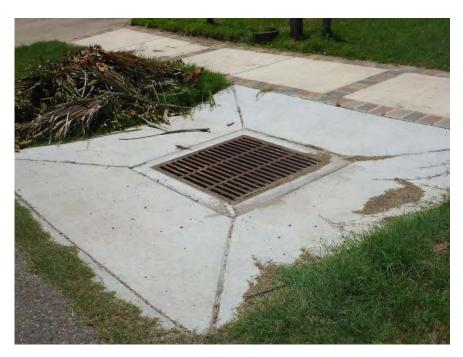
Figure 15. Example Grate Inlet, Laguna Boulevard
