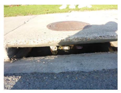
Figure 9. Example Curb Inlet Full of Water and Trash
