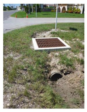
Figure 21. Example Culvert, Laguna Boulevard
