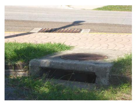
Figure 19. Example Parking Lot Curb and Grate Inlet, Laguna Boulevard
