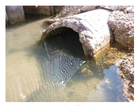
**Figure 8. Example Outfall Degradation**
