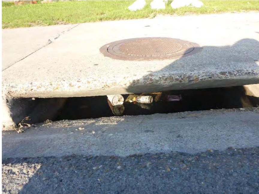
**Figure 9. Example Curb Inlet Full of Water and Trash**
