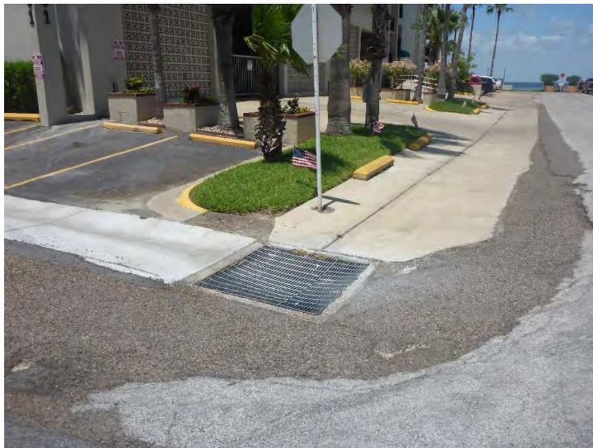
**Figure 16. Example Grate Inlet, Laguna Boulevard**
