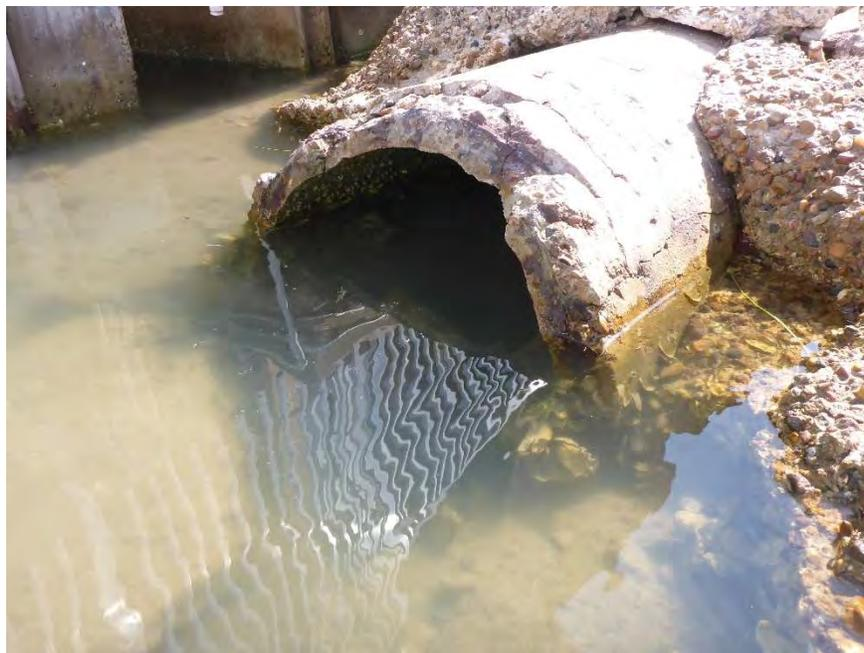
**Figure 8. Example Outfall Degradation**
