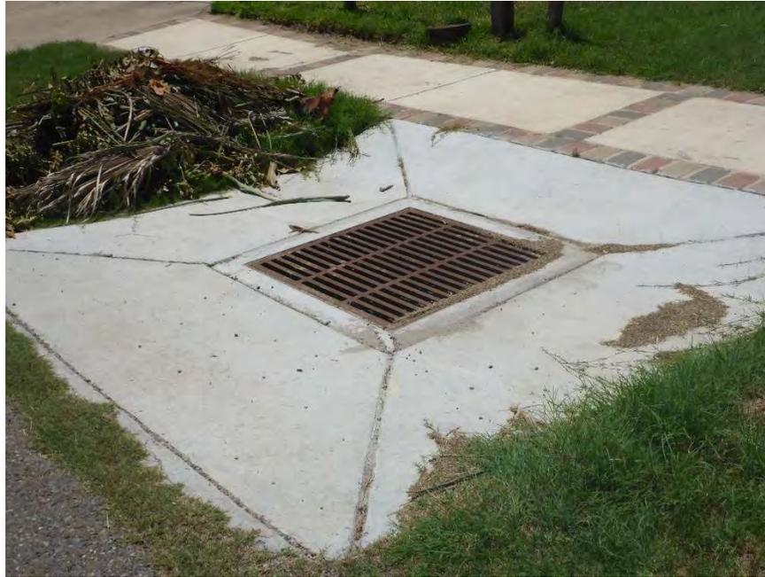
**Figure 15. Example Grate Inlet, Laguna Boulevard**
