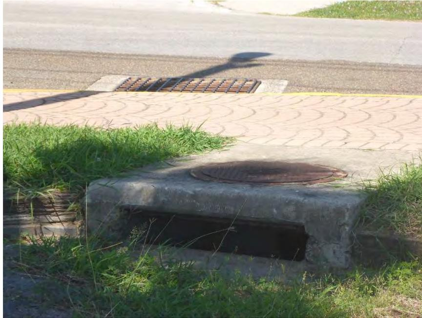
**Figure 19. Example Parking Lot Curb and Grate Inlet, Laguna Boulevard**
