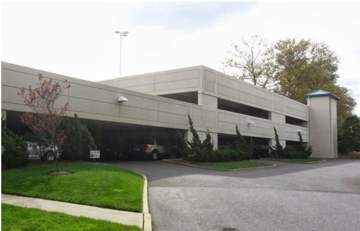
Example of Parking Structure
