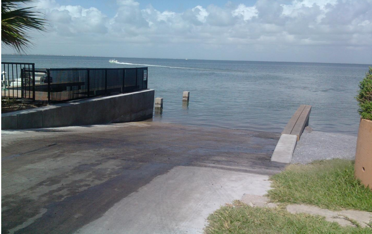
Recently completed Polaris Street Boat Ramp
