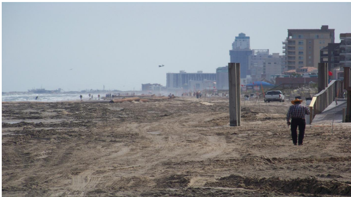
Re-nourishment from dredge material
