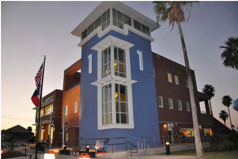
Completed Fire Station
