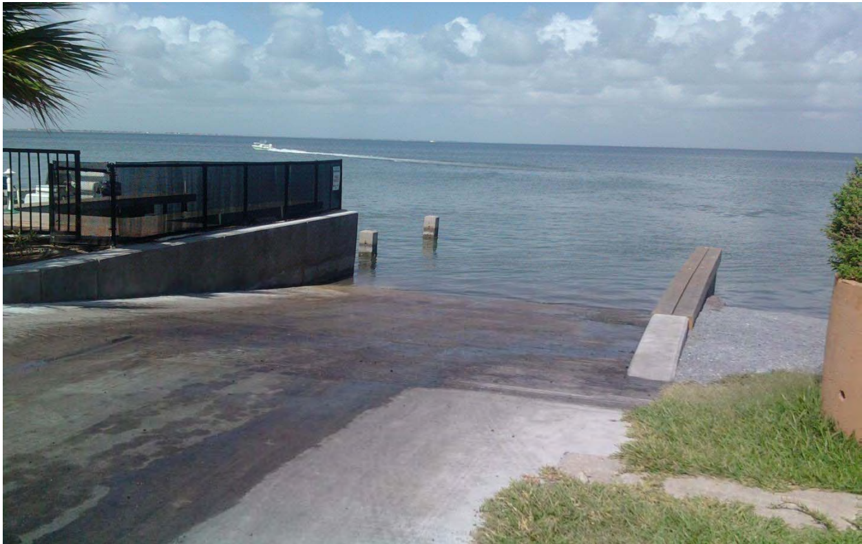
Recently completed Polaris Street Boat Ramp
