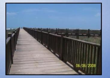
Construction materials: Wood/Trex planking Length: ~ 182 Ft. Width : ~ 6 Ft.
