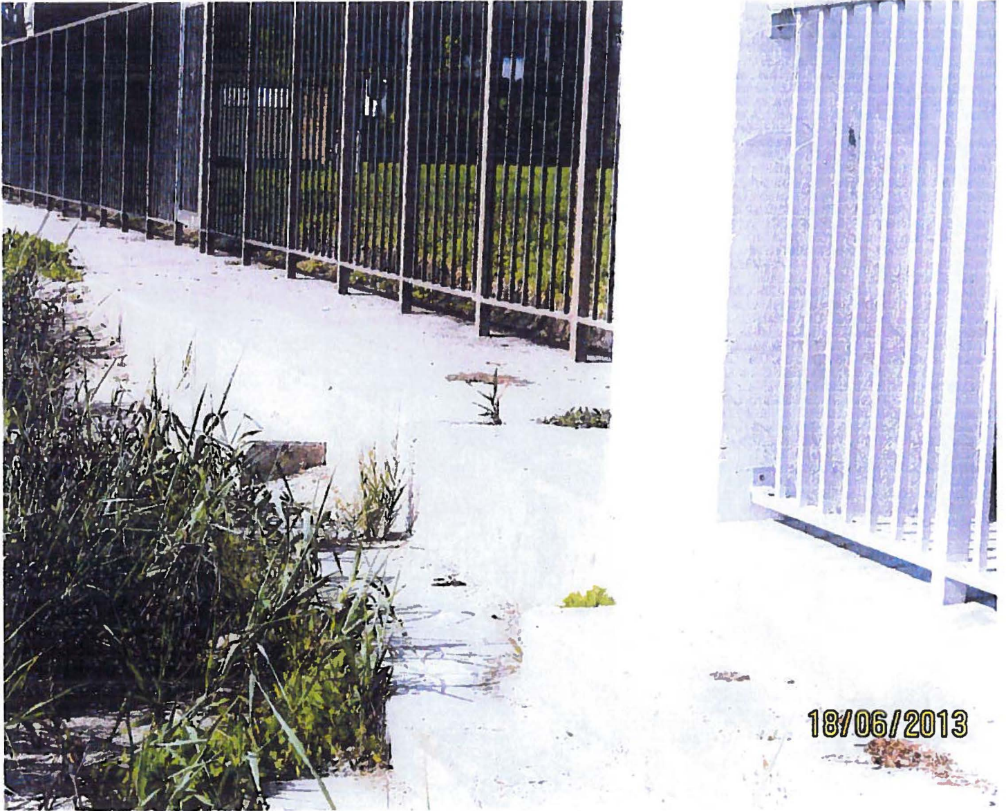
Seawall boundary between Breakers Condos and Isla Del Sol Condos
