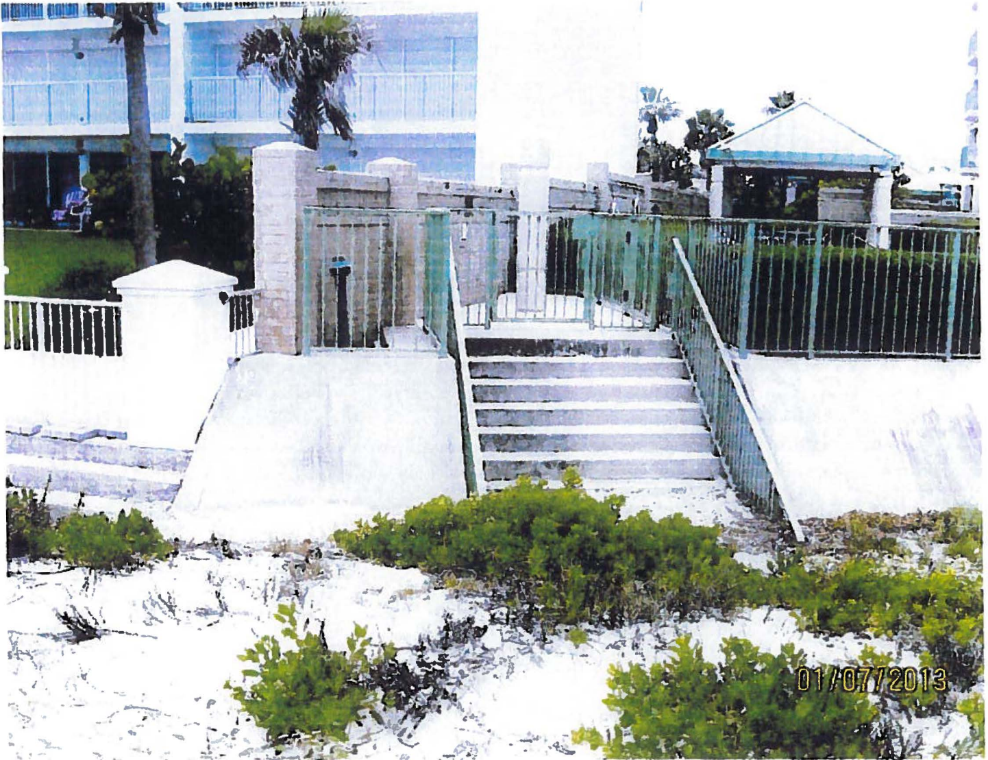
North boundary of Breakers seawall with seawall of Emerald Beach Condominiums
