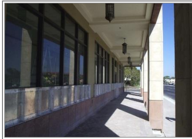
Example of Dry Flood Proofing removable panels utilized in a Bank Building in Naples Fl. – Appropriate in the Bayfront, Entertainment District Core, Neighborhood Crossing, and Town Center Crossing Zones
