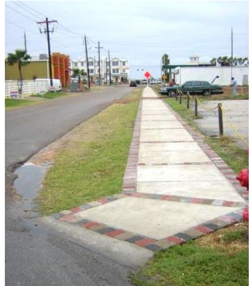
Figure 46 - New Sidewalk Design - Cross Street
