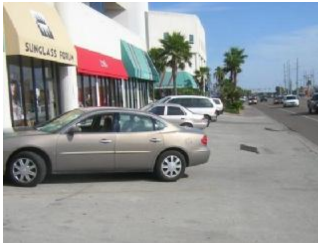
Figure 39 - Pedestrian Path Conditions
