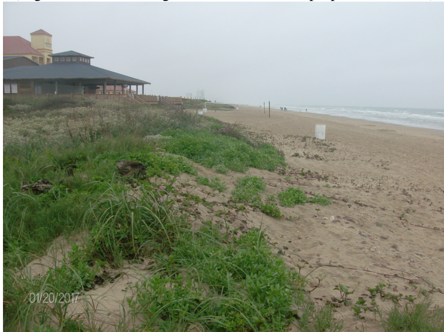
View from the Beach facing north (Gulf of Mexico) These dunes will be built up to elevation 14 and additional Vegetation will be planted
